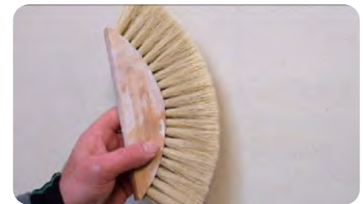
Final phase: brushing the surface (4:15)
