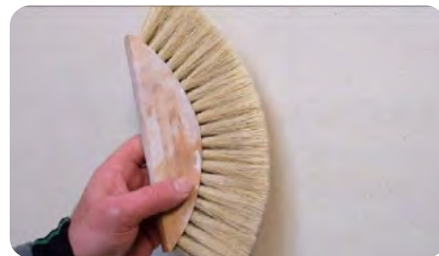
Final phase: brushing the surface (5:00)
