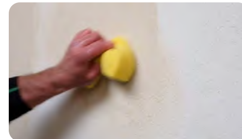
Final phase: wiping the surface (4:00)
