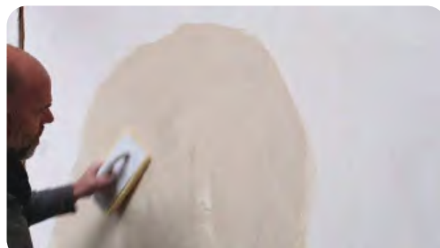
Wiping repaired surface (2:40)
