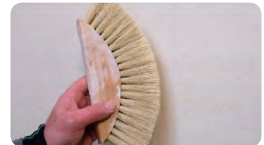
Final phase: brushing the surface (4:30)
