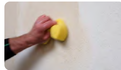
Final phase: wiping the surface (3:40)
