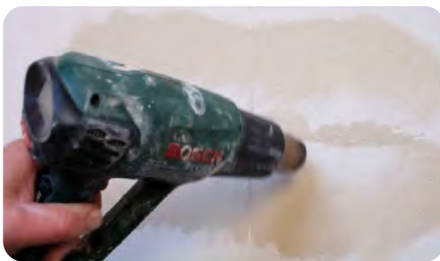
Drying the surface with a heat gun (2:00)
