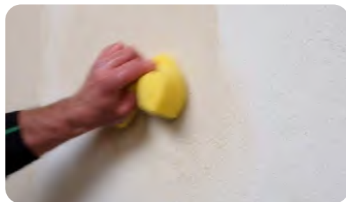
Final phase: wiping the surface (4:45)
