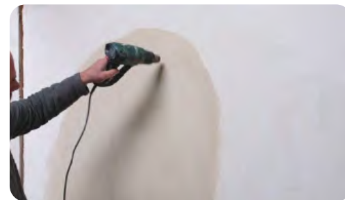
Drying the surface with a heat gun (3:30)
